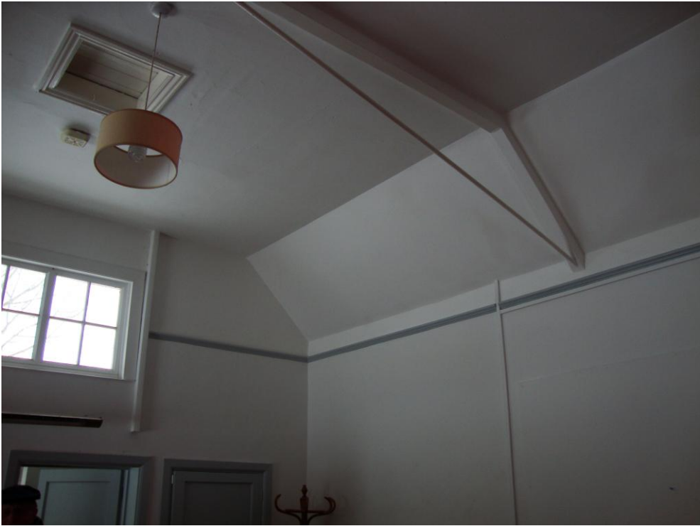
Fig 4: Ceiling of hall showing tie beam, loft access and smoke alarm
