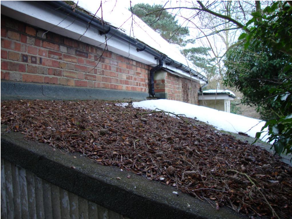
Fig 3: Roof of lean-to
