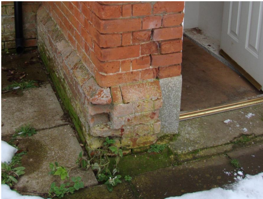
Fig 1: Decay and damp to front wall
