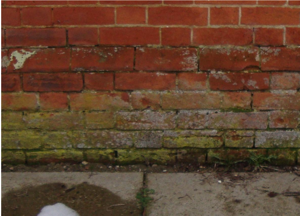
Fig 1: Decay and damp to front wall
